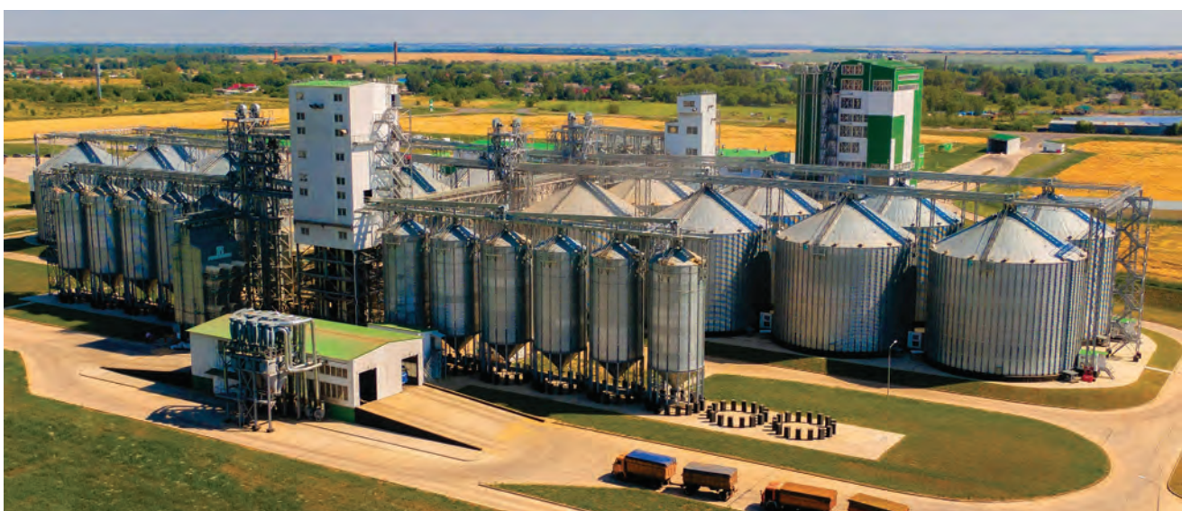
ELEVATOR COMPLEX (COMPOUND FEED MILL) UP TO 127,000 TONS TMK, Tula Region, Kurkino settlement
