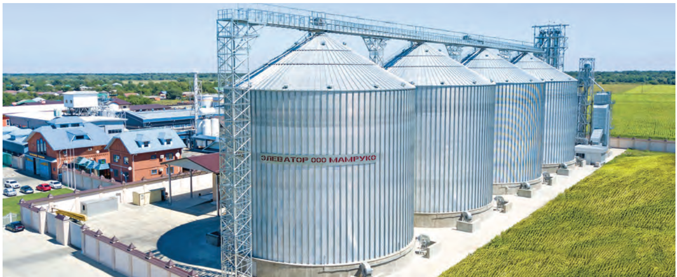
ELEVATOR AT THE OIL MILL UP TO 47,000 TONS Mamruko OOO, Republic of Adygea
