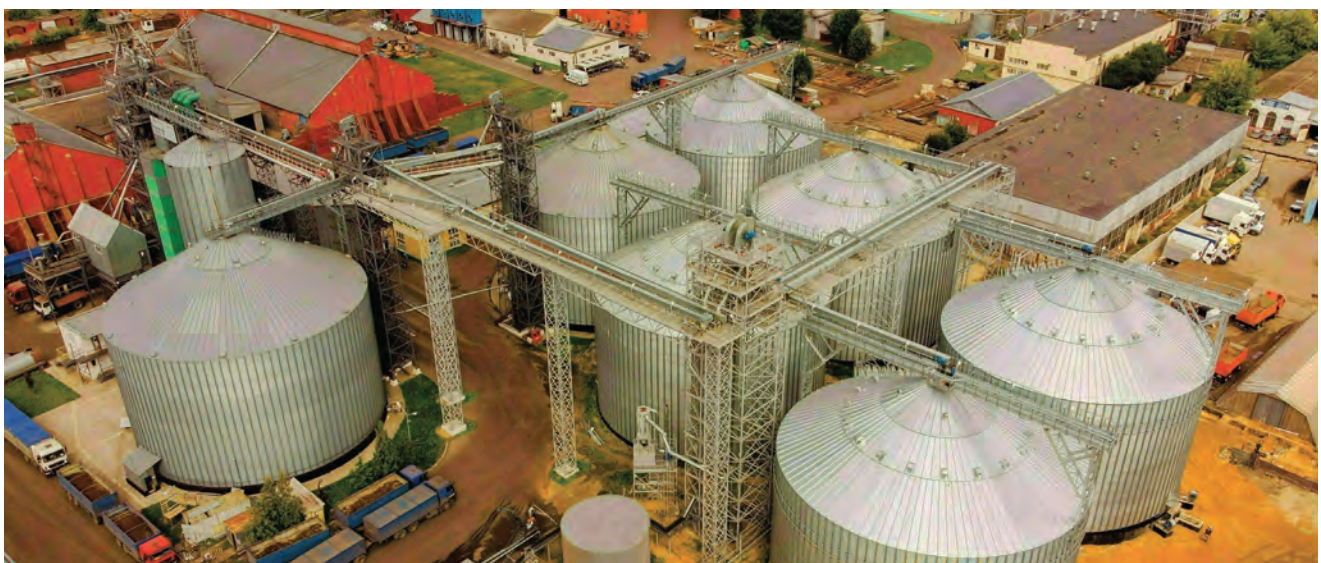
PRODUCTION ELEVATOR (VEGETABLE OILS) UP TO 43,500 TONS Orelstrastmaslo OAO, Orel Region.
