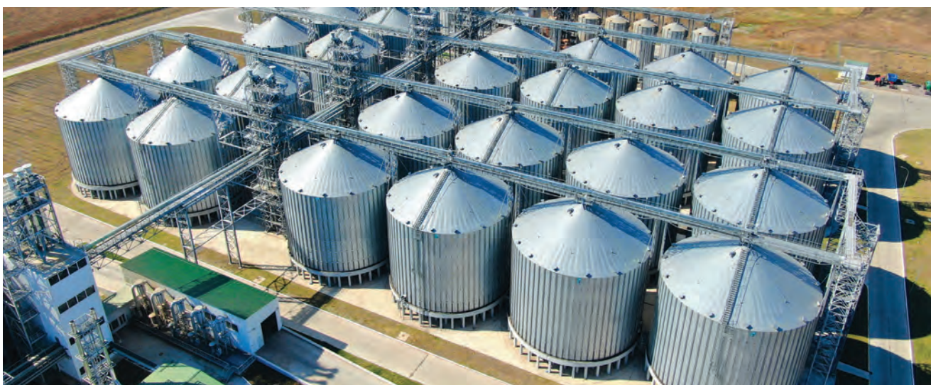
PRODUCTION ELEVATOR (FOR COMPOUND FEEDS) UP TO 130,500 TONS Ecomix GC, Voronezh Region, Pavlovsky district, Gavrilsk settlement
